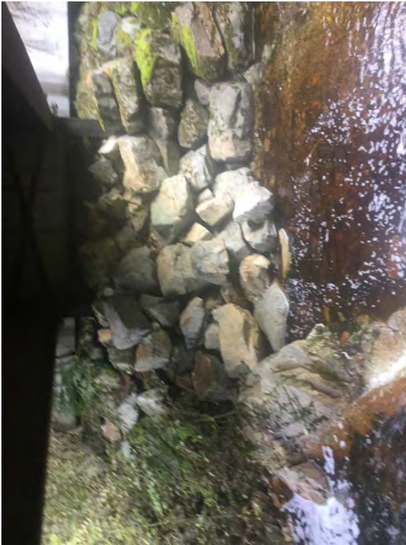
Left Bank Abutment when facing downstream
